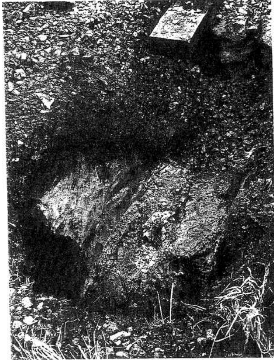
Fig. 5 Cess heave during formation
